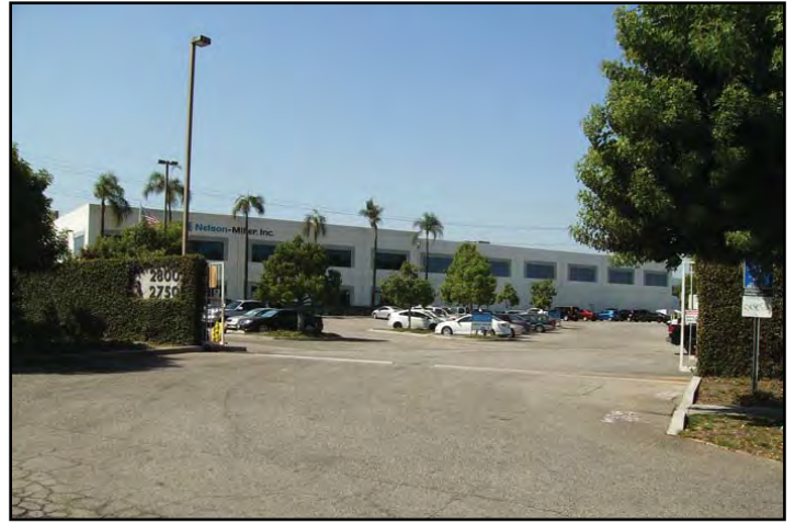
View 2: From the entrance gate to the Project Site, looking southwest at the Project Site.
